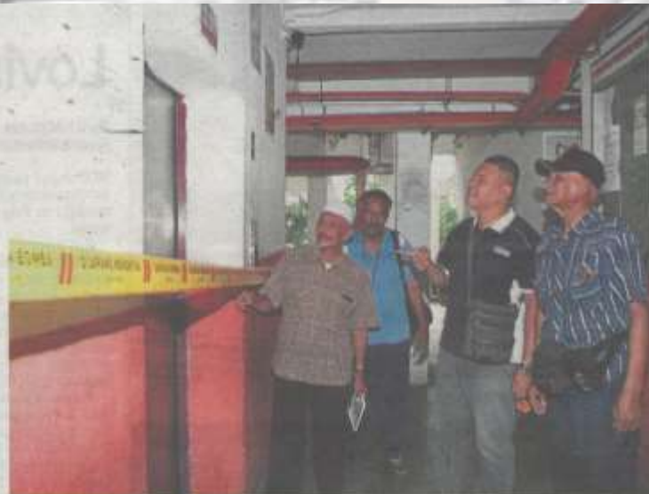
PPR Kerinchi Block C Residents Association chairman Mohd Yusoff Ibrahim (left) with residents of PPR Kerinchi in Kuala Lumpur inspecting the lift which crashed from the fifth floor. — Filepic
