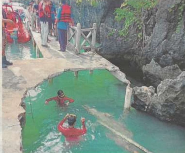
The jetty at Pulau Anak Tikus, Langkawi, which collapsed on Oct 29. Twelve people were injured in the incident. FILE PIC
