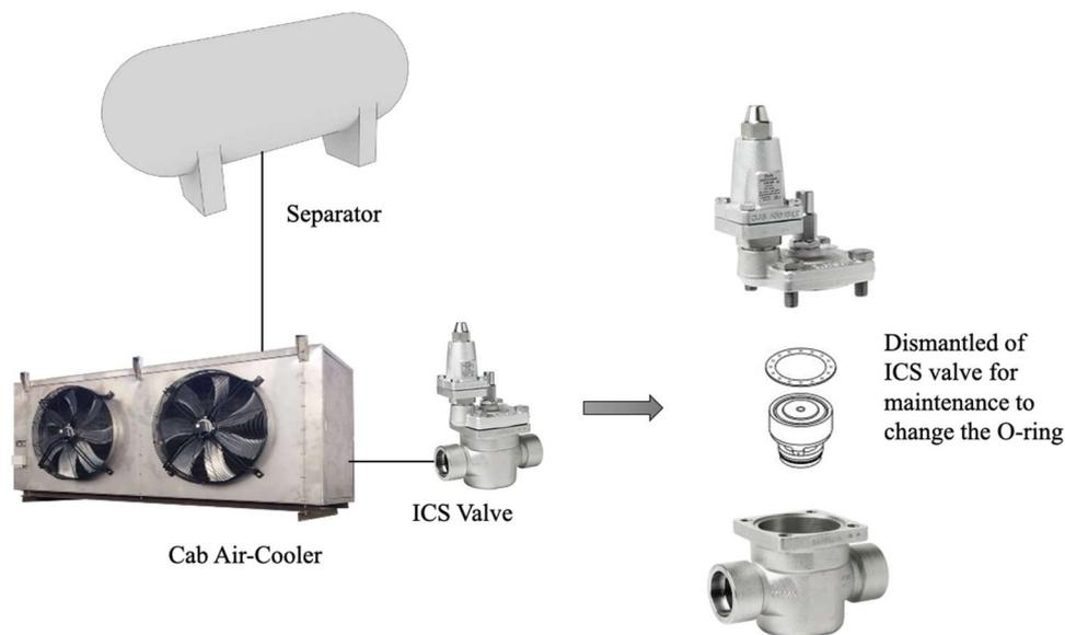
**Figure 13.3.** Dismantling of ICS Valve for O-ring changes at CAB Air Cooler. (Source: DOSH 2020)
