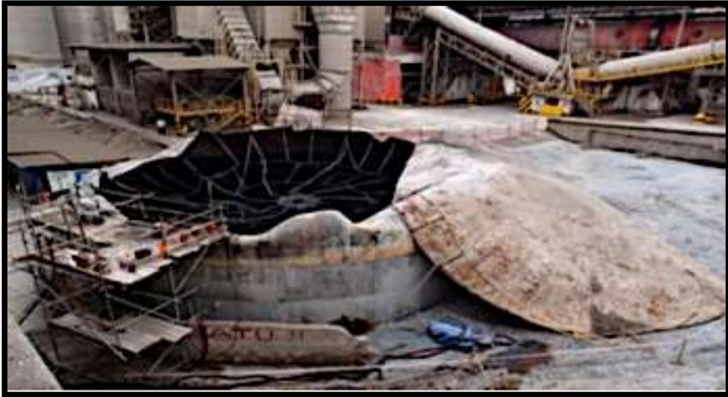
*Figure 10.1. Severe damages on the top and sides of the tank*
