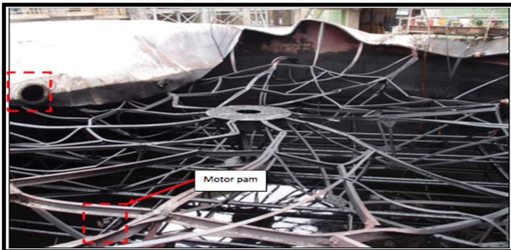
Figure 10.6. Condition of the manhole (maintenance location) and pump motor the remaining RFO
