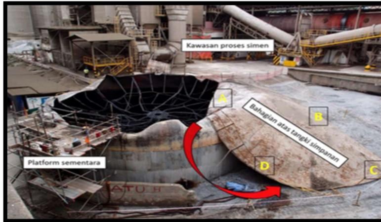
Figure 10.2. The condition of the oil storage tank after the accident
